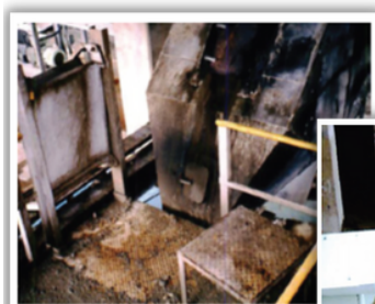
Image 1: Slab box area of the kiln incinerator
